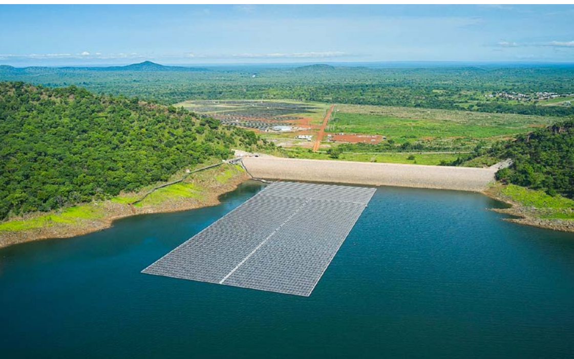
First of its kind in Western Africa, the 5MWp Floating Solar PV System on the Bui reservoir, Ghana.
